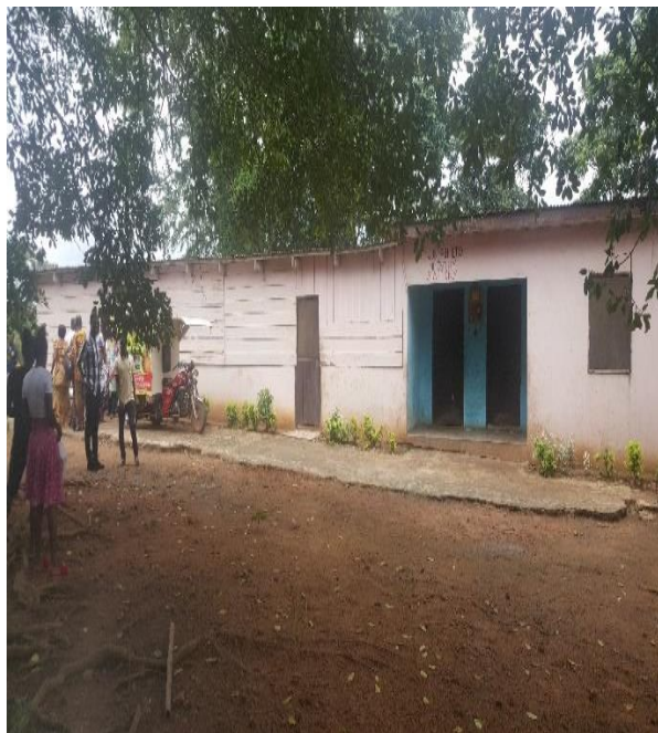
Fig. 3: Local Pumpkin Processing Factory
