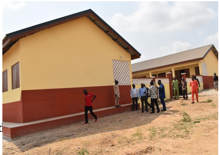
AFRANCHO CLASSROOM BLOCK
