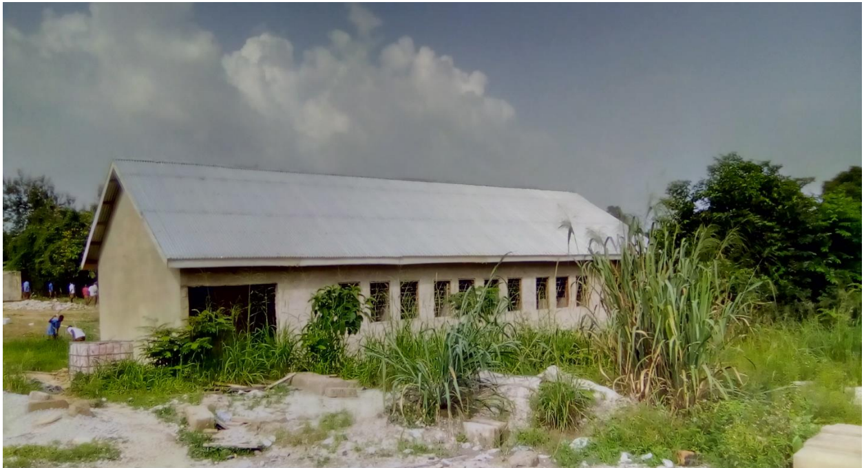
ADUMAN SHS WC
